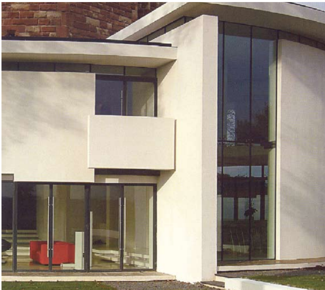
Lymm Water Tower, Cheshire Architect and building owner – Ellis Williams. System designer – Alumasc Exterior Building Products Ltd. Installer – Pegasus Externals Ltd.
