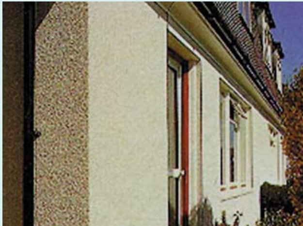
Figure 16 Example of a refurbished low-rise building
