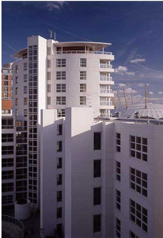
EWI system supplied by weber building solutions, architects: Goddard Manton, photography: Brauer Associates
